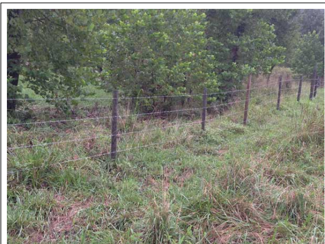
Bison fencing does not have to be like Jurassic park. Most of our fencing is simply 4 strands of barbed wire. Periphery fencing is 5 strands and in vulnerable areas, we add two strands of electric.
